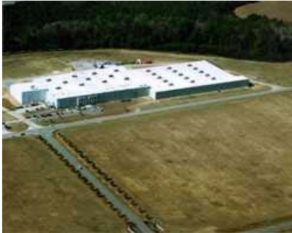
Pictured above: Chicken of the Sea - Georgia Canning facility located in Lyons, Georgia
